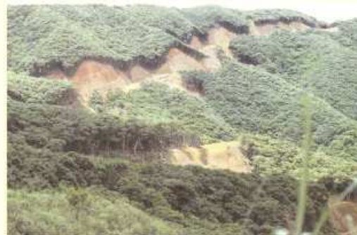
イタジキ林を切りひらいて進む大規模林道工事 Okuni Forest Road construction in Itajiki forest.
